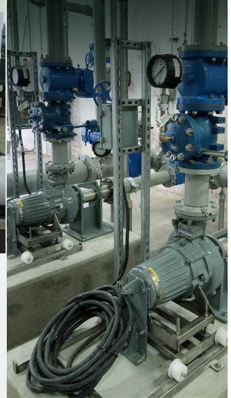
Two alternating Flygt pumps with service carts and telescoping inlet.
