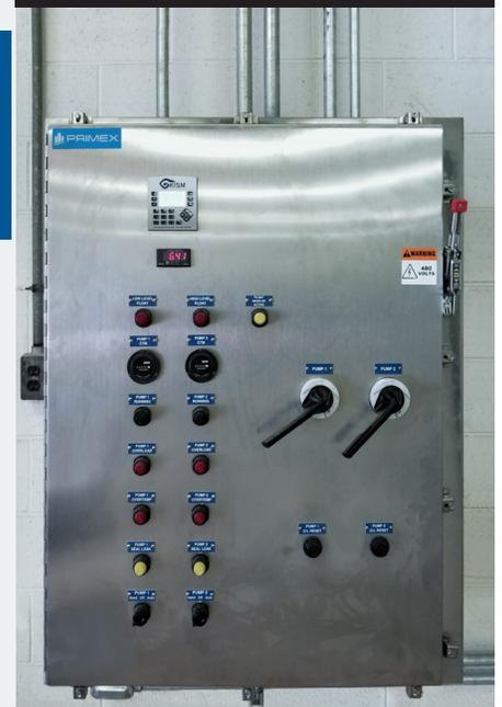
Custom control panel to regulate two alternating Flygt pumps and the equalization tank inlet valve.
