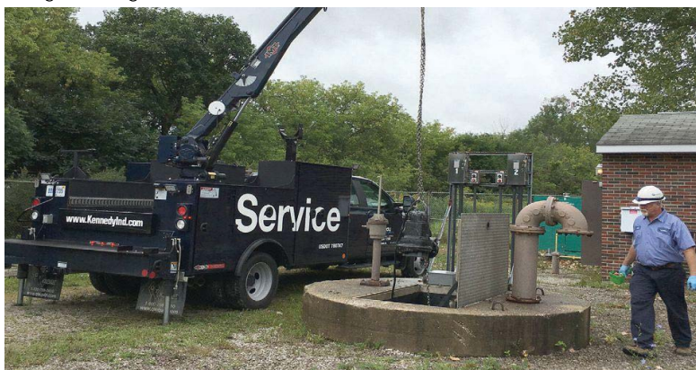
Removal of old pump from Station #8
