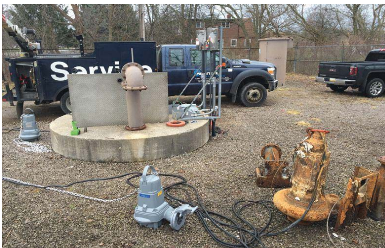
Two new Flygt Concertor pumps being prepared for installation
