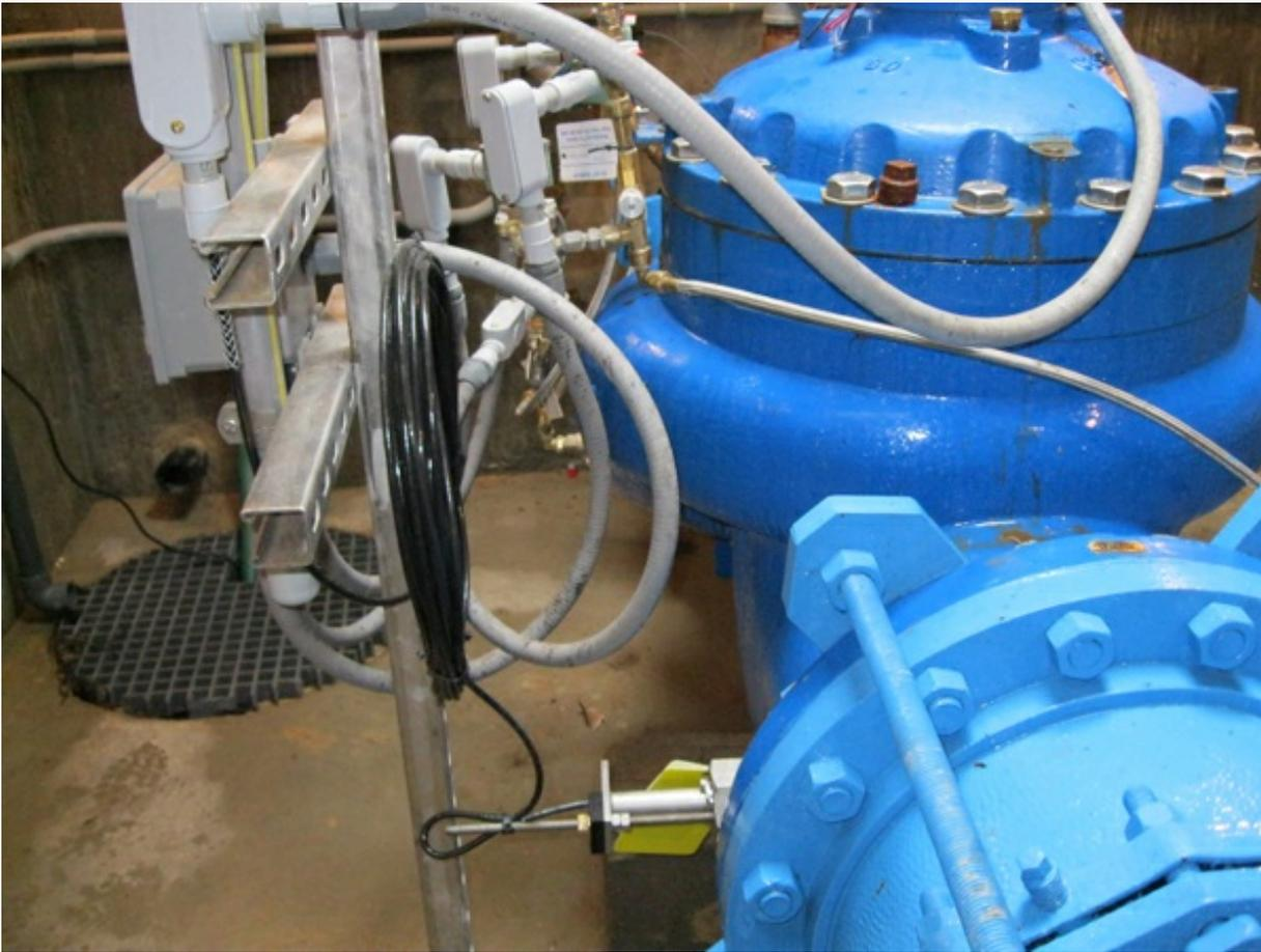
PRV with two pressure-reducing pilot controls. (Courtesy Singer Valve)
