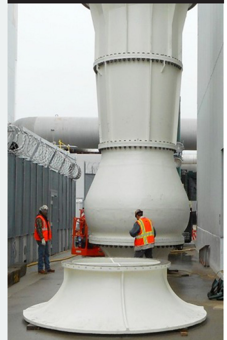
After being assembled outside pump is being lifted to install in pump basin
