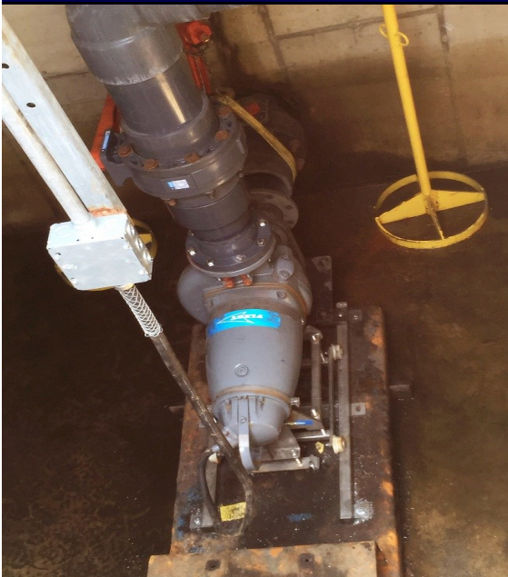
FLYGT SUBMERSIBLE DRY PIT IS FLOOD PROOF
