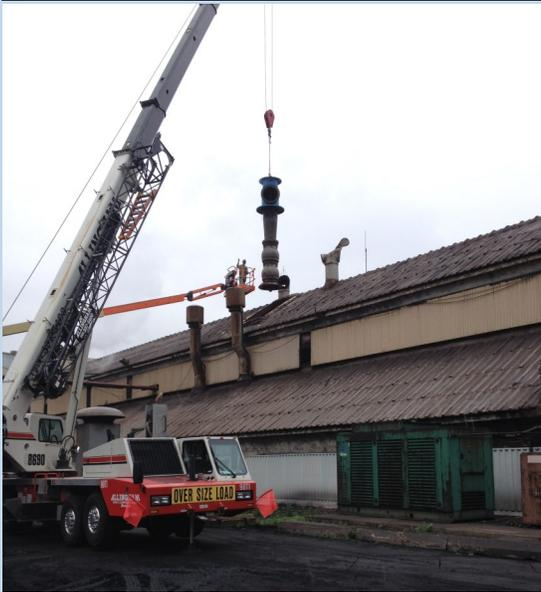
**Problem:** Mill Water Pump #7 was originally purchased as an emergency Y2K pump. However, the pump wasn't installed until several years later. When the pump was finally put into service it was discovered that the motor thrust bearing was undersized and could only last 1,500-2,000 hours. Installing a large thrust bearing in the motor was cost prohibitive, the pump was seldom in operation and only used in emergency situations.
