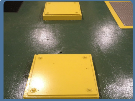
Cover plates replaced motors
