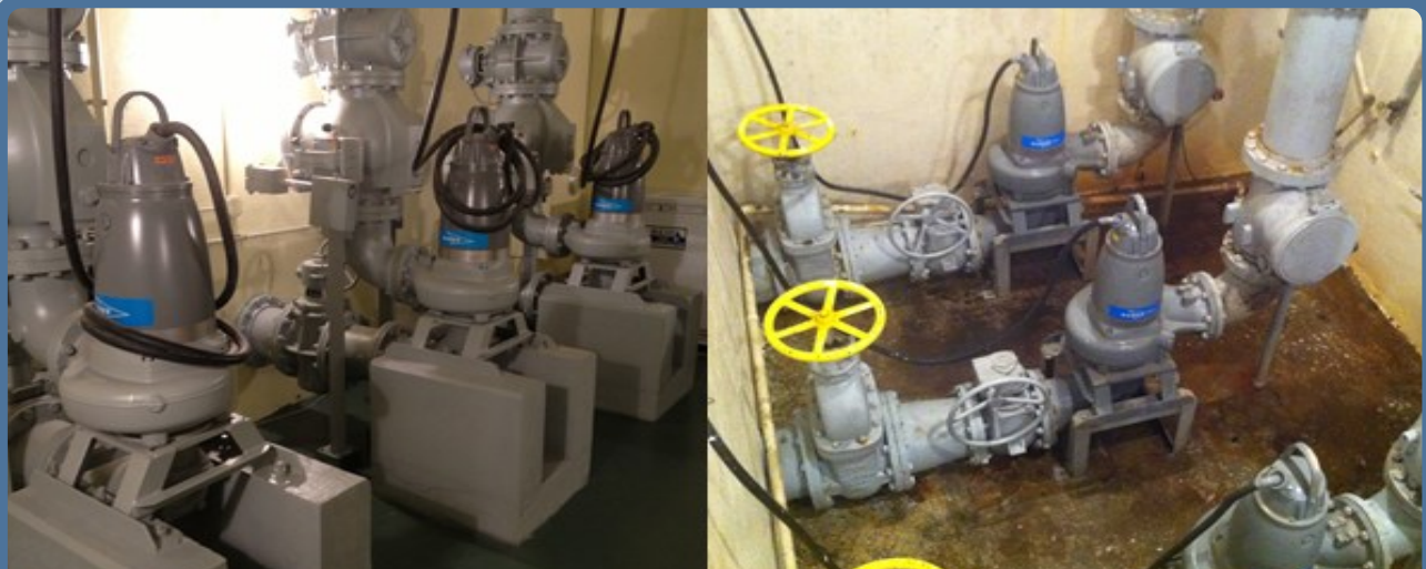
Flygt dry pit submersible pumps provide quiet, reliable, cool running, safe and efficient operation for peace of mind
