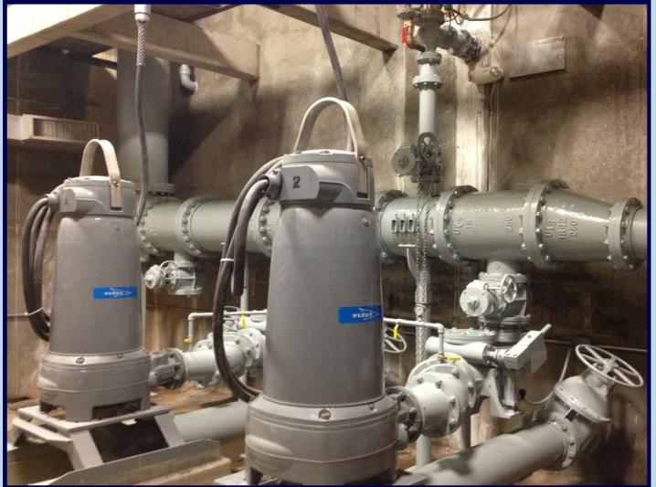
Standard air cushioned check valves and ITT Pumpsmart VFD's allowed for the elimination of the old style hydraulic oil operated valves decreasing complexity of the system.
