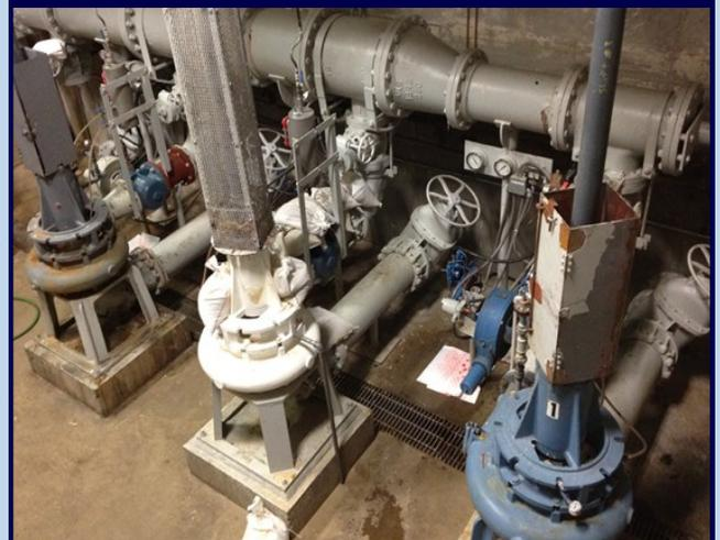
Shafting, coupling guards, seal system, compressor, bearings and hydraulically operated valves required constant maintenance and repair
