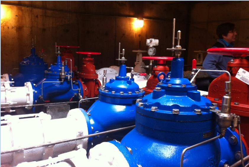
**Two 10" and two 8" Singer Pressure Reducing Valves installed in Bloomfield Township's Inkster Vault**
