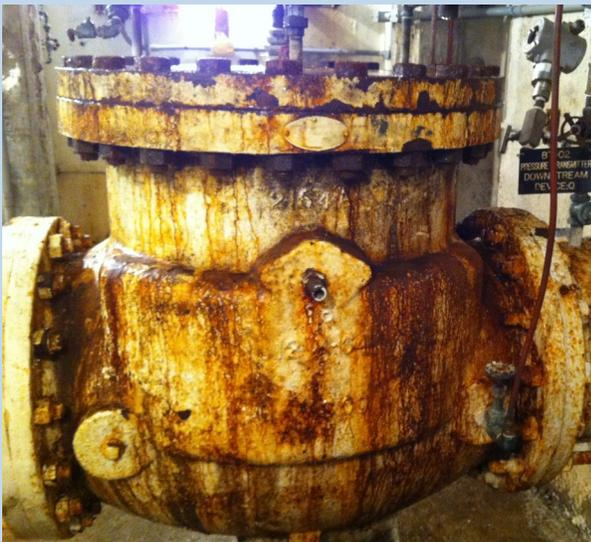
Existing PRVs performed inconsistently and were difficult and expensive to repair
