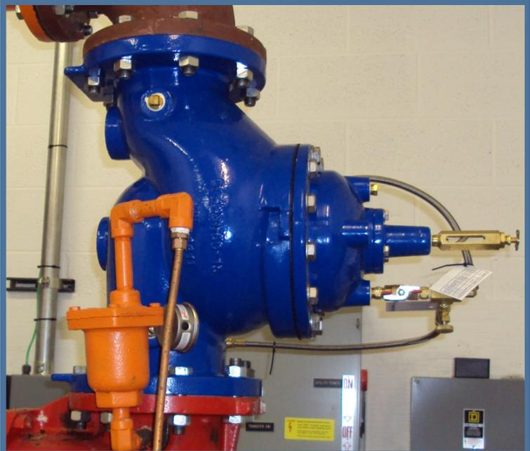
**New Singer Pressure Relief Valve installed at the Country Creek Station**
