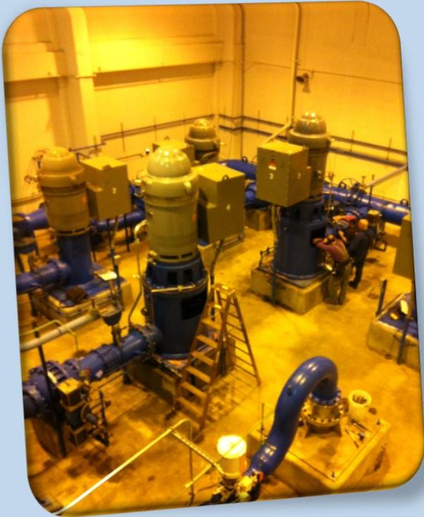
**PROBLEM:** A large Mid-Michigan Chemical Company was replacing old, outdated, and, inefficient fluid drives on 500 HP vertical turbine pumps. The pumps are located at a local municipality water plant and provide critical cooling and process water to the chemical plant.
