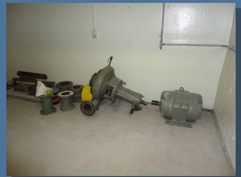
WYMAN'S PRE-EXISTING PUMP AFTER REMOVAL (RIGHT)
