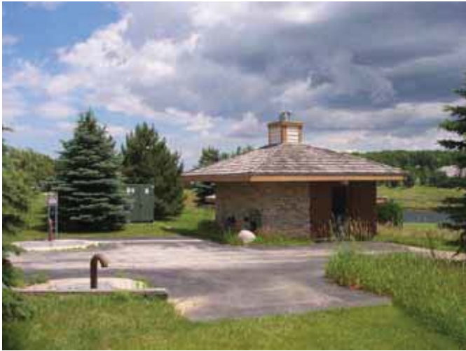
By switching to a different type of pump, the Village of Hartland, Wis., eliminated frequent clogs and reduced energy consumption at the Arlene Drive Lift Station by more than 60%. Jim Fischer
