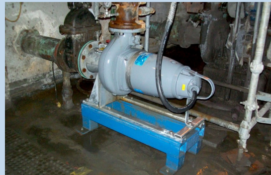
NEW FLYGT PUMP WITH HIGH CHROME IMPELLER
