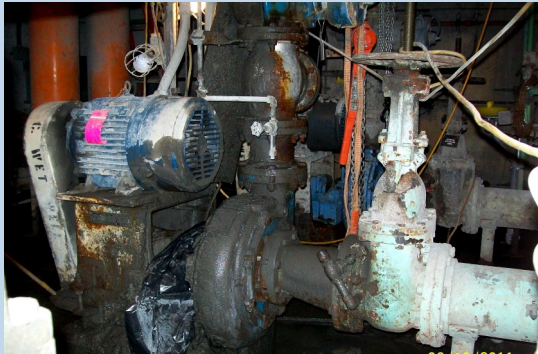
EXISTING PUMP PRIOR TO REPLACEMENT
