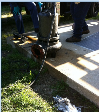
Competitor pump being unclogged
