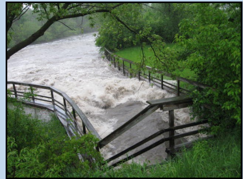
Allen Creek Drain surging during a storm.
